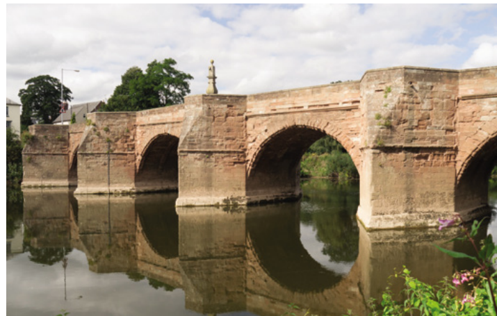
Wilton Bridge, Ross on Wye
