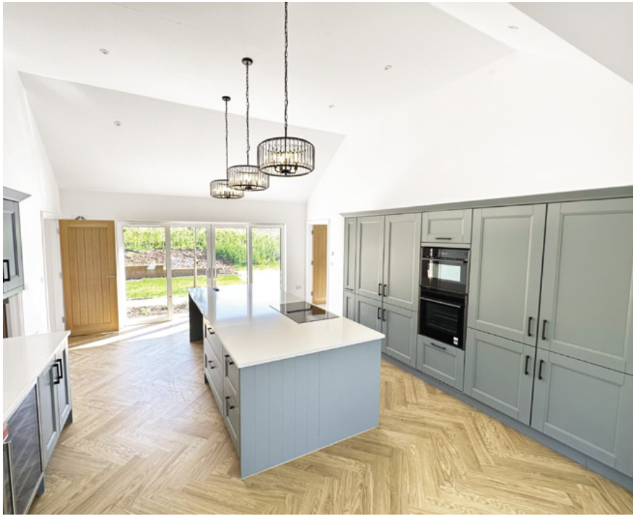
Full height ceiling to kitchen
